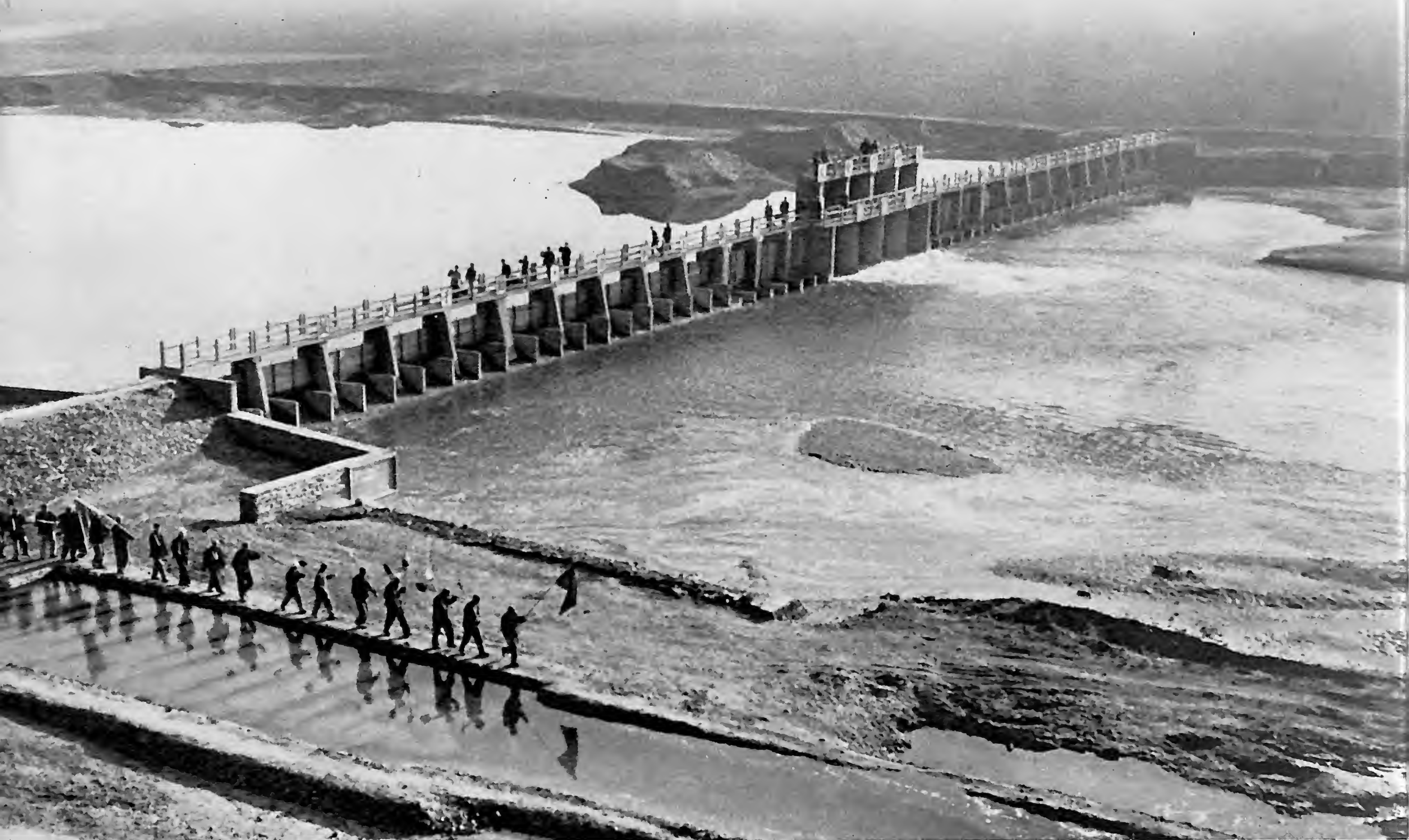
This dam 114 metres in length built by the members of Tangchih commune, Yingkou County, makes it possible to bring 6,000 mu of cultivated land under gravity irrigation. Maintaining the spirit of self-reliance, commune members throughout Liaoning Province have completed a number of small reservoirs, dams, wells and other projects.
